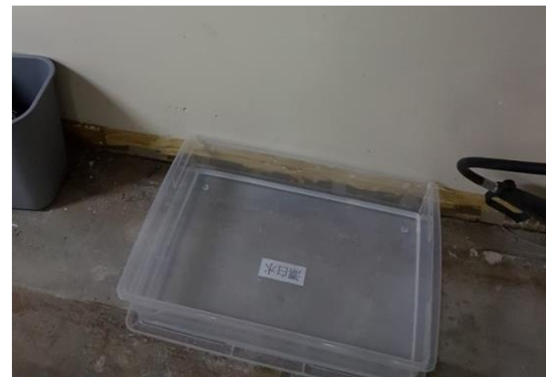
Shoes washing basin with disinfection liquid for before site leaving to prevent dust be taken from shoes
